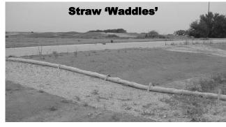
Ground covers can slow the flow of water reducing erosion and allowing sediment to settle out.
