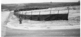
Properly located and installed silt fences can greatly reduce the amount of sediment that leaves a construction site.
